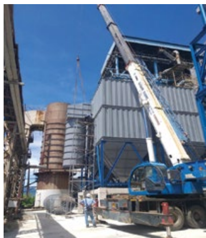
The boiler has been renovated at Ninh Hoa - Bien Hoa Sugar factory
